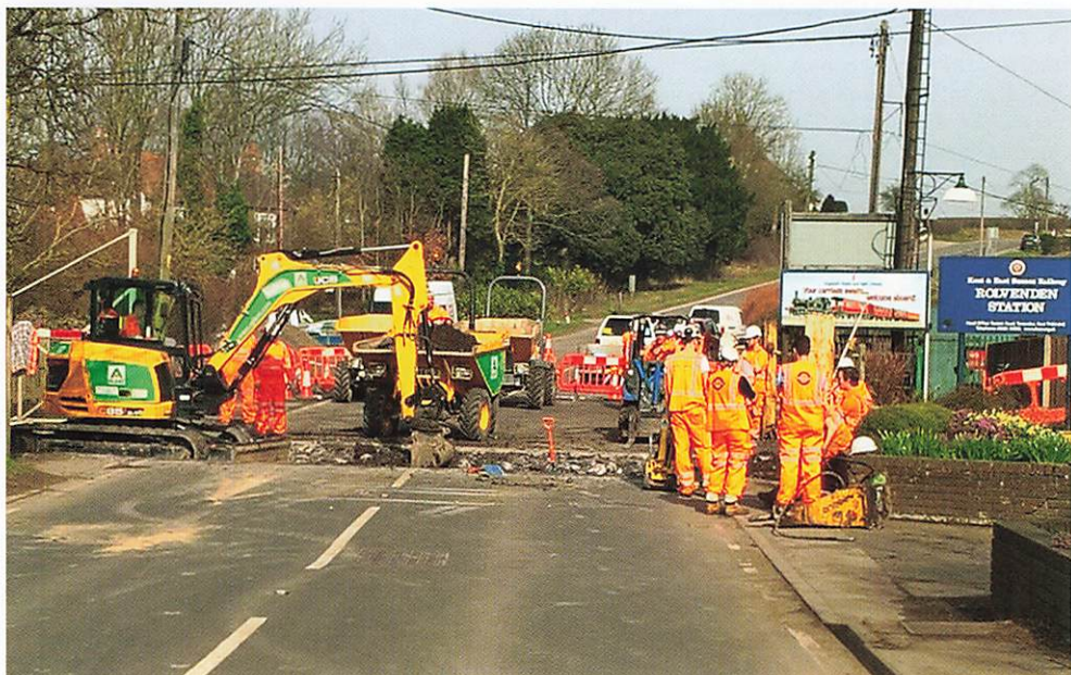
Breaking out the old crossing.
