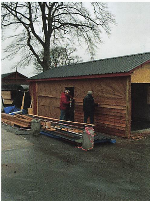
Installing the cladding.
