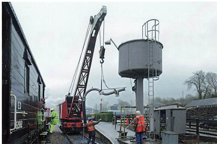
Refitting the arm to the water crane at Northiam on 1st March.
