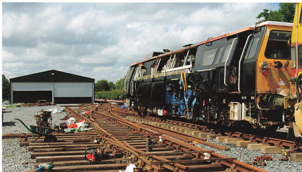
Midsummer view south of the new carriage storage shed. Note the double-slip turnout under construction.
