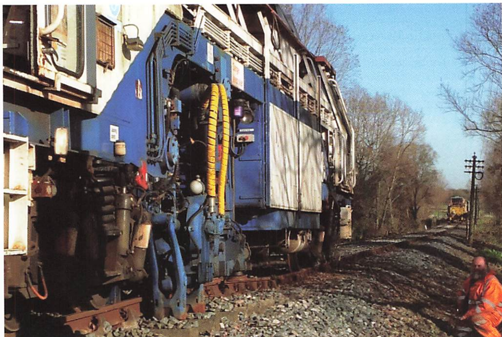
Volunteer Frim Halliwell views the position of the Tamper's tines during PWay work at Hexden Bridge (Jamie Douglas)
