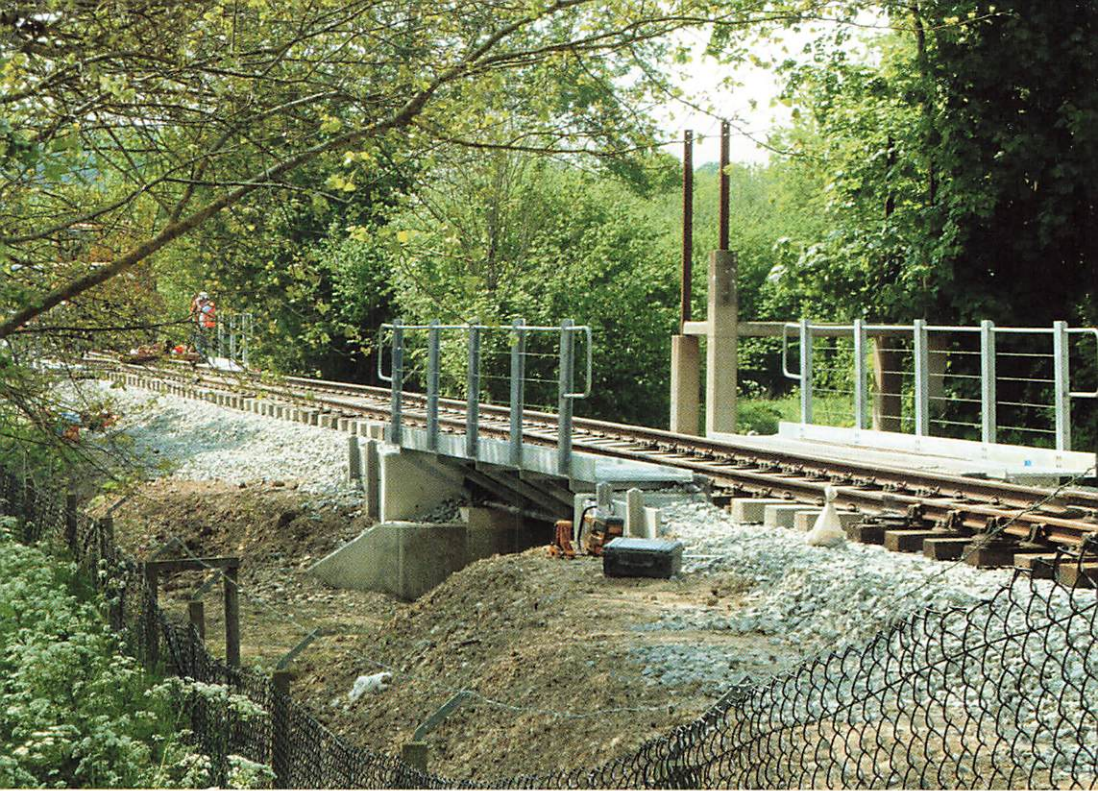
Track being laid over bridge No. 5 at Robertsbridge (Mark Yonge)
