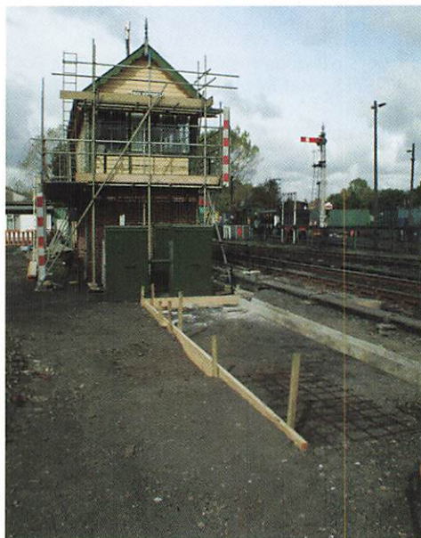
Rolvenden Box shrouded in scaffolding ready for painting; note base for new signalling relay room being prepared in front (Paul Wilson)
