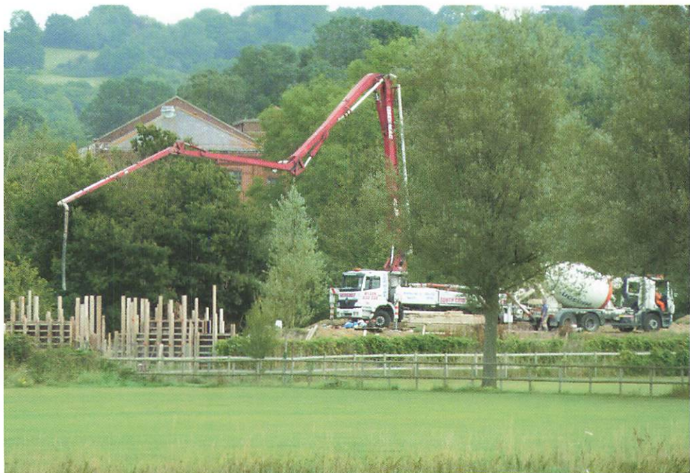
The concrete pump from South Coast Pumping. Its 34m reach is evident and is the only way to actually do the pour simply (Duncan Buchanan)
