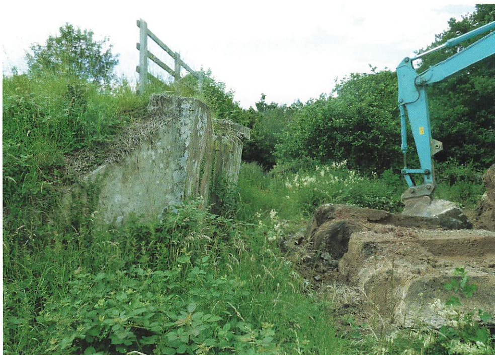
Bridge 3 in early stages of demolition; note left hand side leaning inwards abutment, these were not secured to the other side and thus floated on a sea of clay (Duncan Buchanan)
