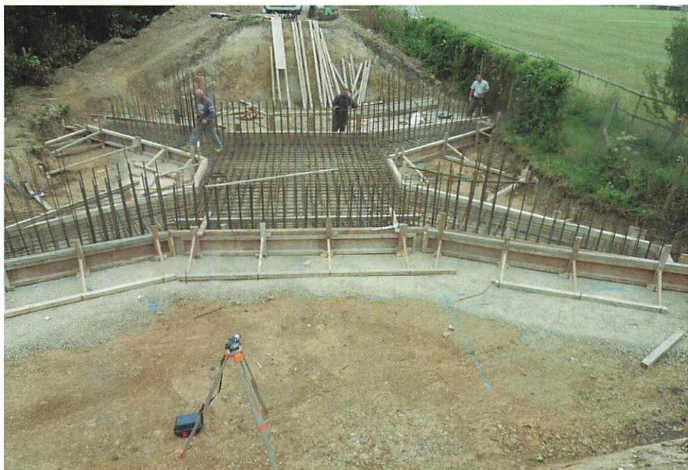
DDF sorting out the reinforcing before the first pour; note the upright rods are ready for the walls and a later concrete pour (Duncan Buchanan)
