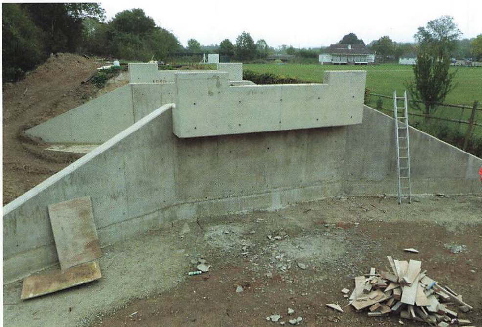
The completed Bridge 3; only needs bridge span and backfilling of the embankment to finish off a clean job (Duncan Buchanan)
