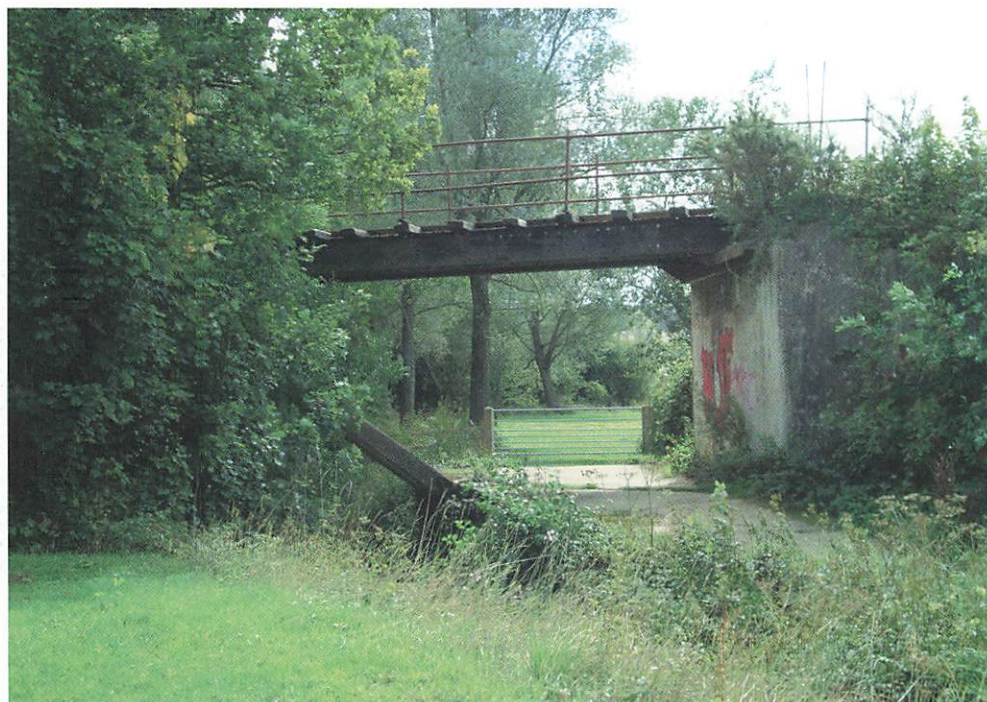
Bridge No. 1 outside Robertsbridge. Note concrete prop to allow for failed invert (Mark Yonge)
