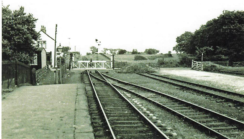
Eastchurch station and level crossing, not long before closure. The road to the left led to the aerodrome. Note the mound of earth serving as a buffer stop (via Tom Burnham)
