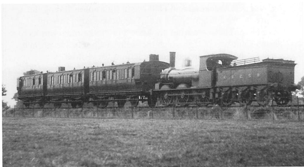
K&ESR ex GER coaches set pulled by No.7 Rother approaching Headcorn; acetylene light fittings visible on roofs of all three carriages. August 1910
