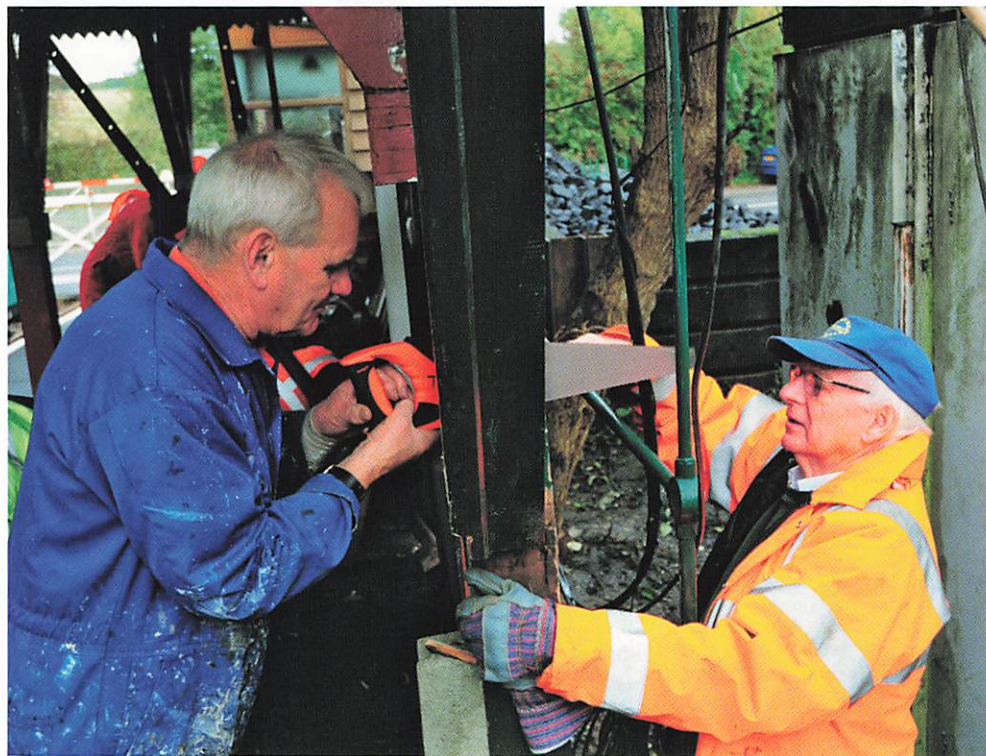
Ron Dunn and Norman Bourden cutting out rotten wood on Rolvenden canopy upright (John Rose)
