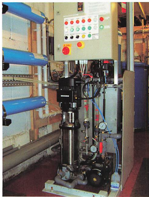
Reverse Osmosis plant, underneath the water tower at Rolvenden. (Chris Greatley)
