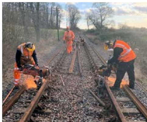
Clive Fitzjohn and Dave Latham cut rails to length under the watchful eye of Mike Popperwell.
